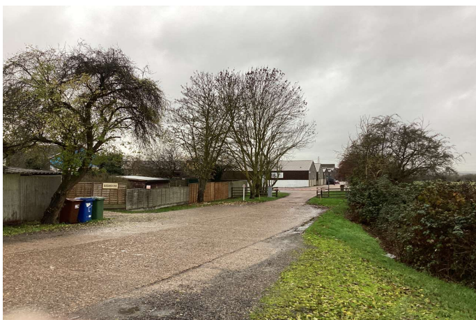
Looking south-west from the north-west corner onto agricultural buildings.
