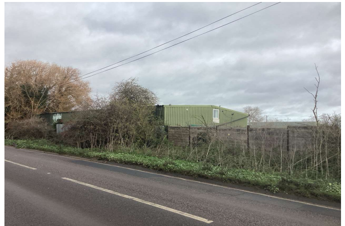
Looking west from the east onto a warehouse unit.
