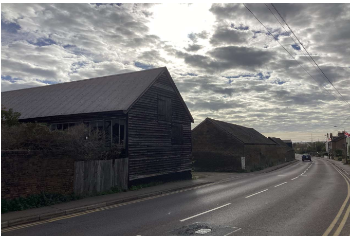
Looking south-east from the north-west corner across Ship Lane onto farm buildings along the boundary of the sub-area.
