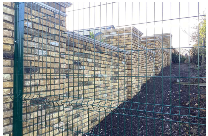
Looking east at the north-east corner at the brick wall on the north boundary.
