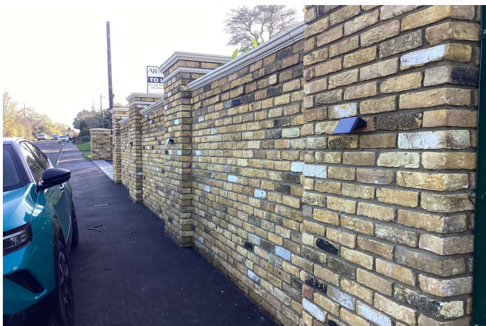
Looking south from the north-east corner at the brick wall on the east boundary
