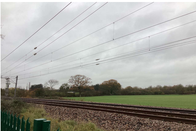
Looking south-west from near the south corner onto the railway line and field.
