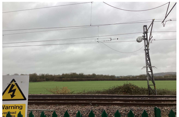
Looking north from near the south corner onto the railway line and open field.
