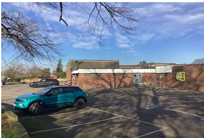
Looking north-east from the west boundary at a carpark and country club building.
