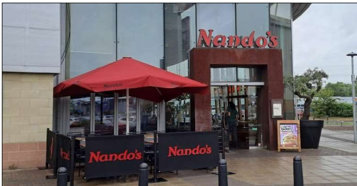
Figure 9: Nando's, Lakeside Retail Park
