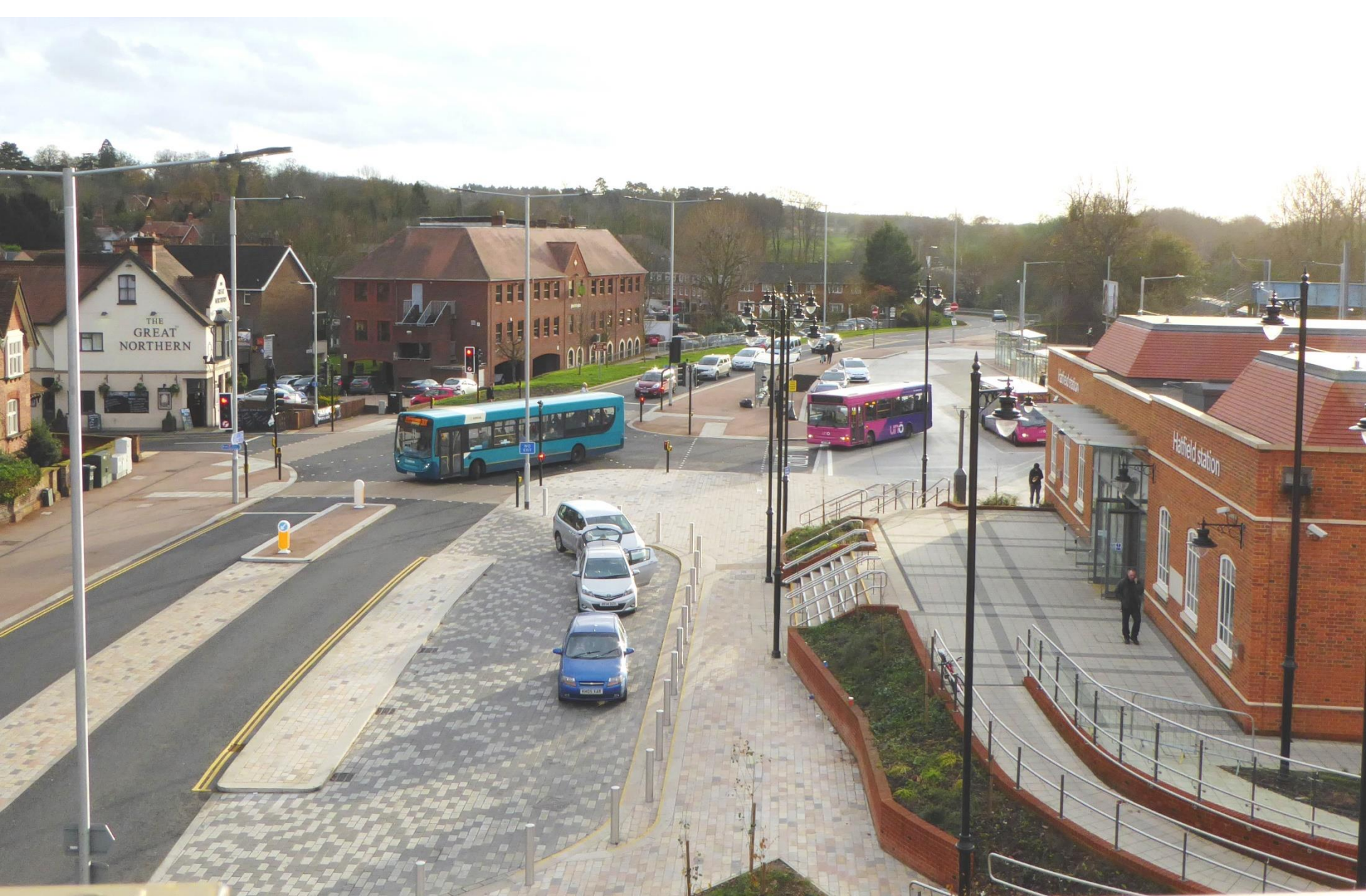
A1000, The Great North Road – after upgrade, speeds slowed, courtesy crossings, high quality public realm
