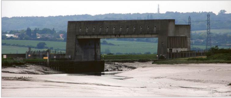
Figure 5-1 Fobbing Horse Tidal Barrier (Source: South Essex CFMP) 29
