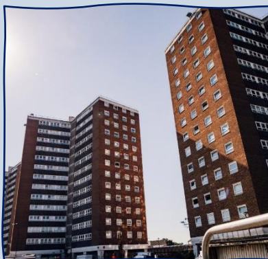
© Chadwell St Mary's Retrofit Project (Kensa, 2023)
