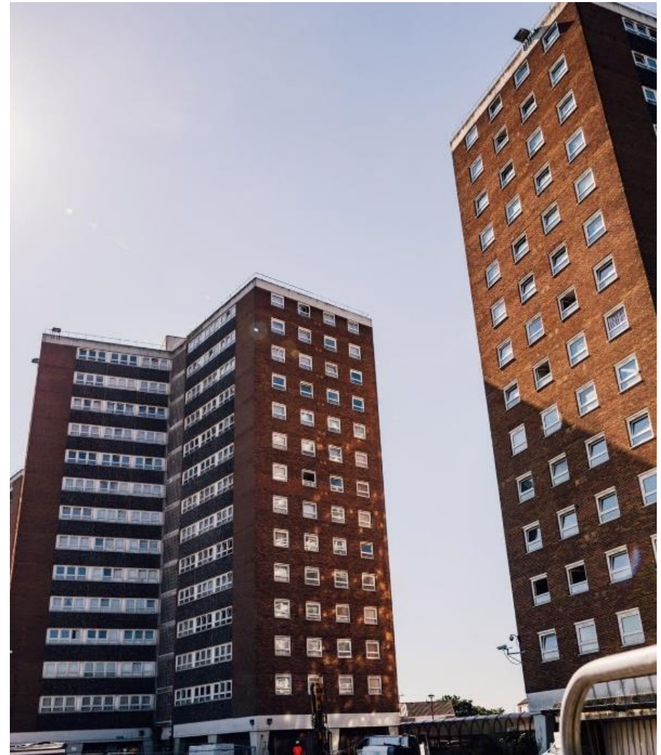
© Chadwell St Mary's Retrofit Project (Kensa, 2023)
