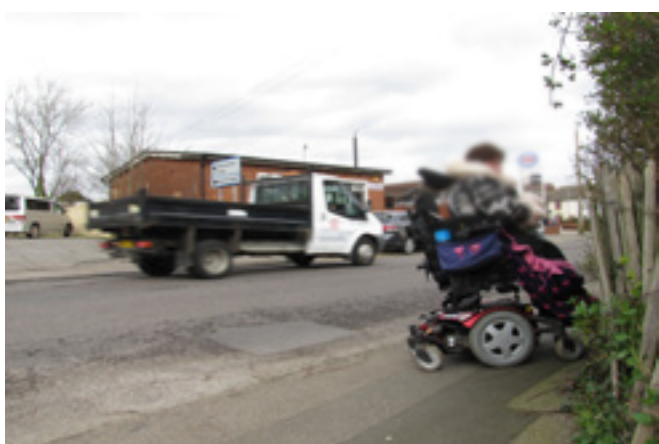
Dangerously steep cross falls across pavements
