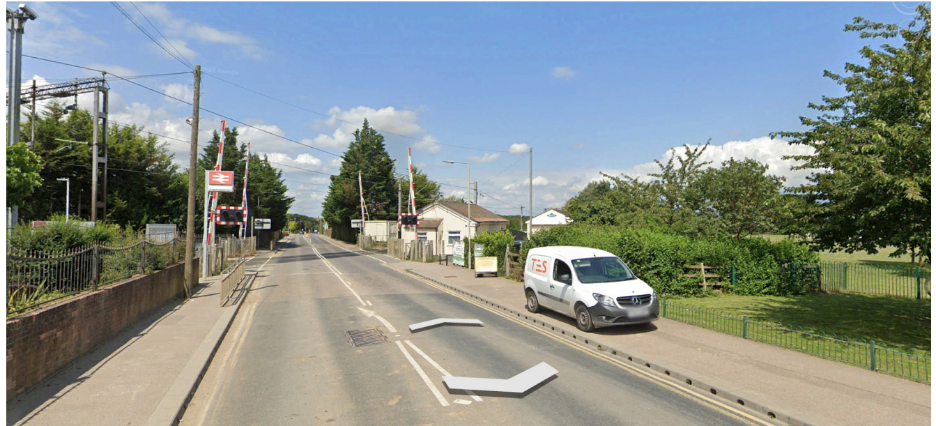
Level crossing with Gobions Park to the left
