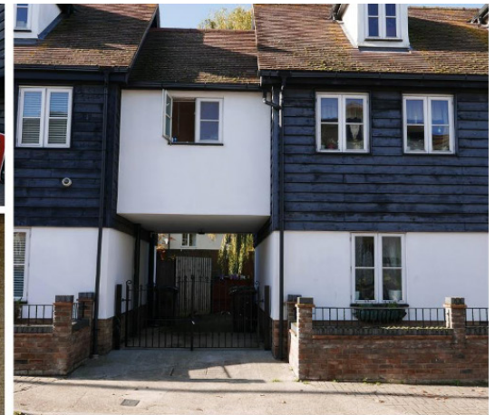
Parking tucked behind housing, also a common feature in nearby Orsett.
