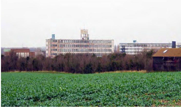
The Bata Factory, East Tilbury, the former factory complex of the British Bata Shoe Company.
