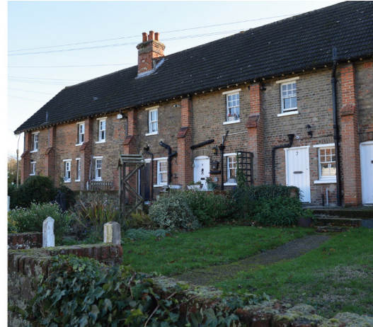
Workers cottages in a terrace with a simple brick palette, which continues into the garden steps and walls.
