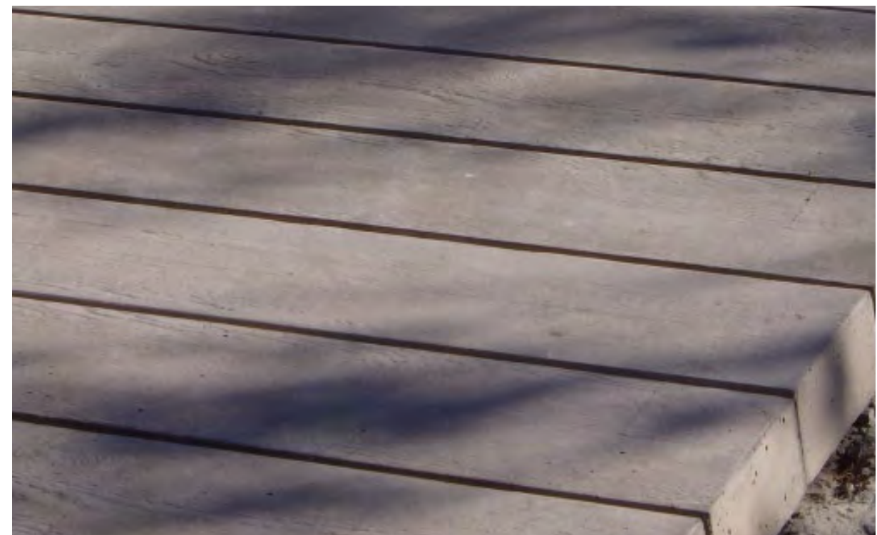
Example of precast concrete boardwalk with a cast-in form liner finish that provides a long-term, anti-slip solution
