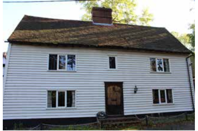
Figure 26: Numbers 1 and 2 Hall Farm Cottages (Grade II Listed 1111621)
