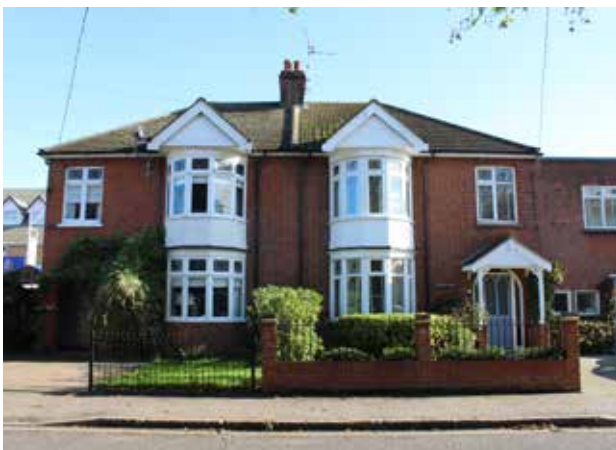
Figure 86: Two dwellings showing the impact of alterations. Window replacements, concrete roof tiles, porch and a garage extension have affected character.
