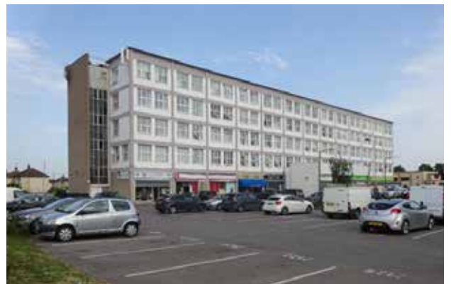
Figure 30: Car Park at Stamford House
