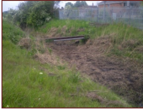
FIGURE 4: EAST DOCK SEWER AFTER VEGETATION CLEARANCE
