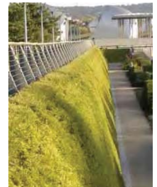
Thames Barrier Park, London, UK
