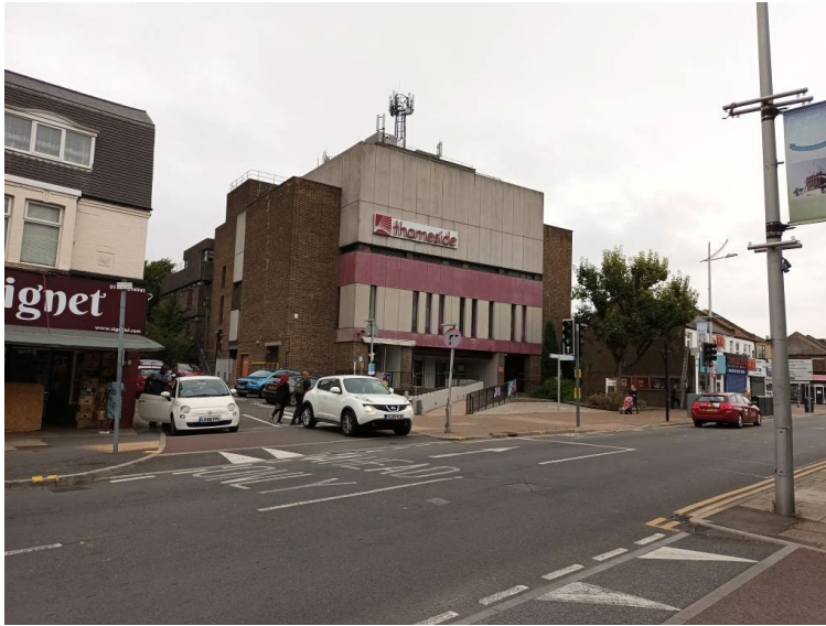
Figure 5.9: Grays Town Centre: Thameside Complex
