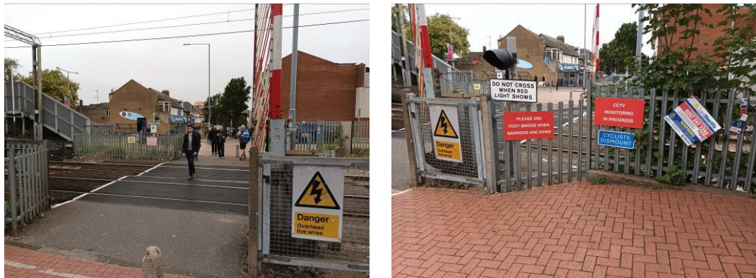
Figure 5.26: Grays Town Centre: Level Crossing
