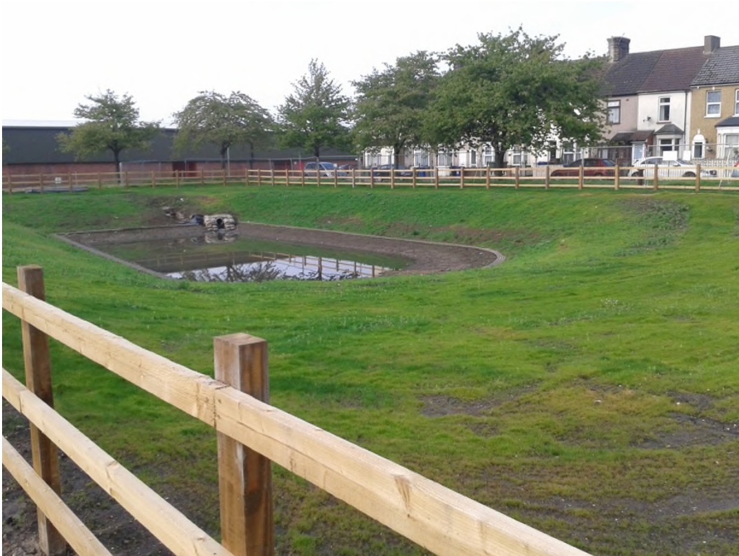
Figure 1: Drainage Pond at Gumley Road
