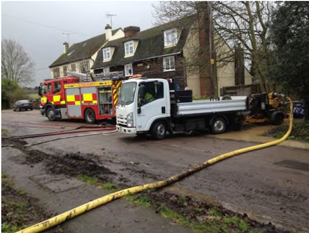
Figure 2: Emergency pumping of flood water
