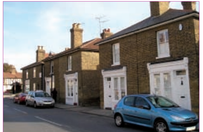
High Road (south side)
