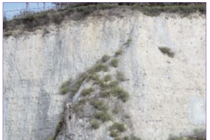
Chalk cliff face under Tank Lane
