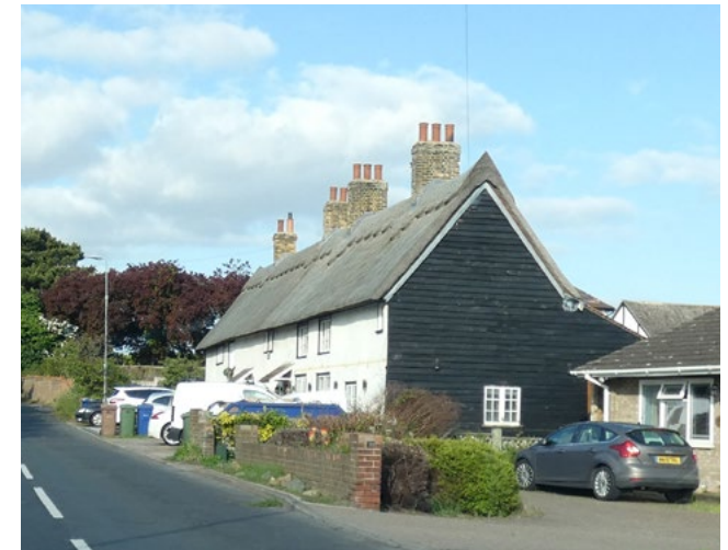
Fig 56. c17 Listed Building Slades Hold Cottages
