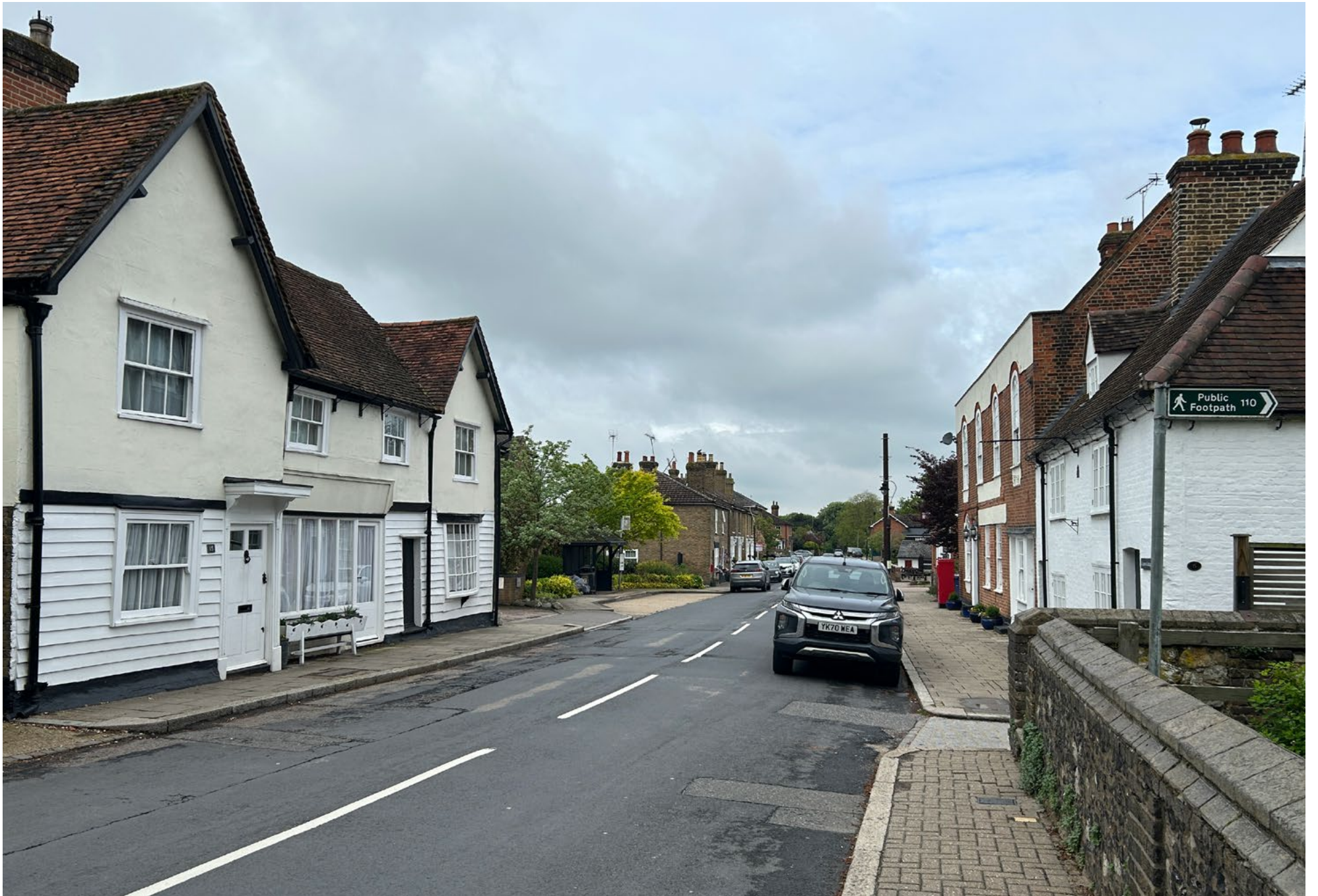
Fig. 32 Orsett High Road, facing west
