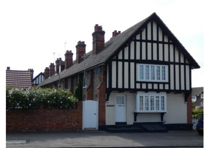
Fig 82. Former Maltings that is of Local Heritage Interest
