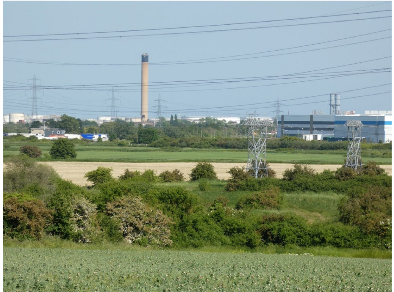
Fig. 38 Division A looking southwards from Viewpoint 1 over former marsh-land towards Coryton and London Gateway.
