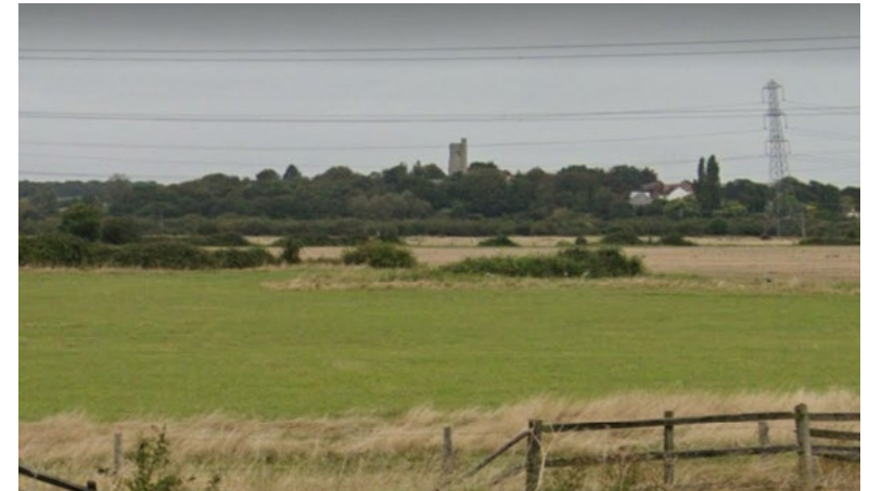
Fig 52. Grade I listed St Michaels Church, looking north from Viewpoint 2 on the A1014. Image from Google Streetview (Oct 2021)
