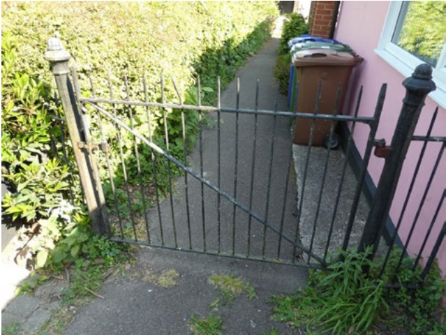
Fig. 34 Cast Iron rear gate to Grade 1 St Michael's Church
