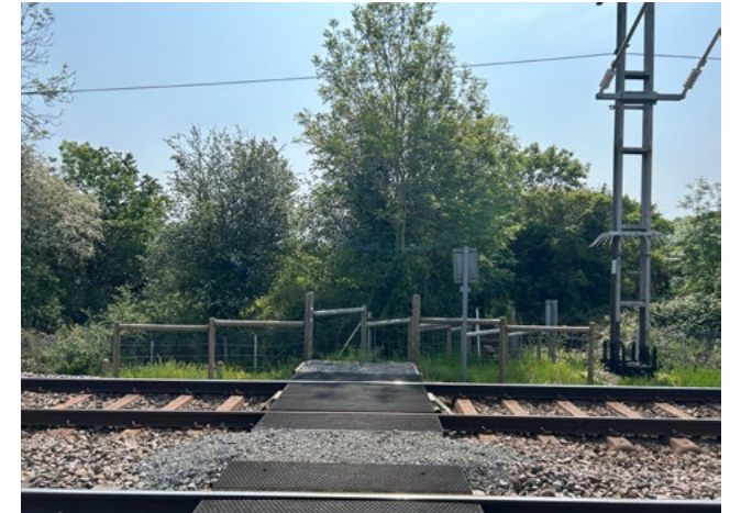
Fig 83. Footpath 23 crossing the railway
