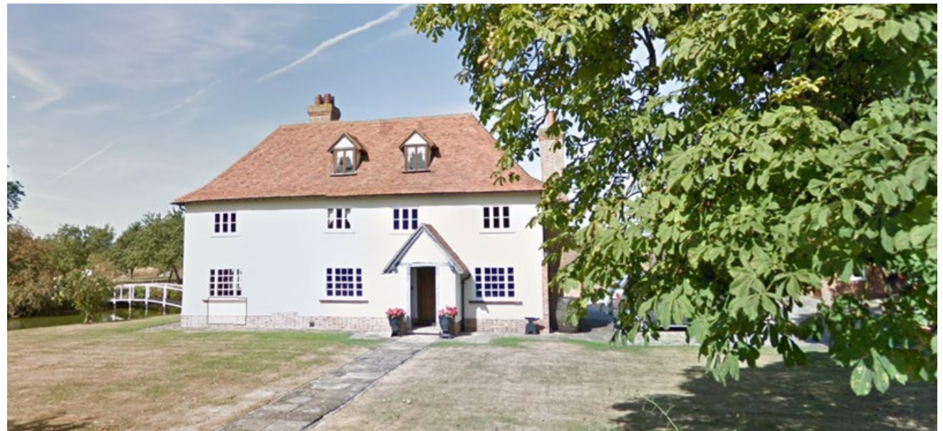
Fig 56. Grade II listed c16 Garlesters - image from Google Streetview dated Sept 2016
