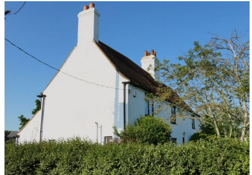
Fig. 49 Grade II listed Slough House commands the setting of China Lane
