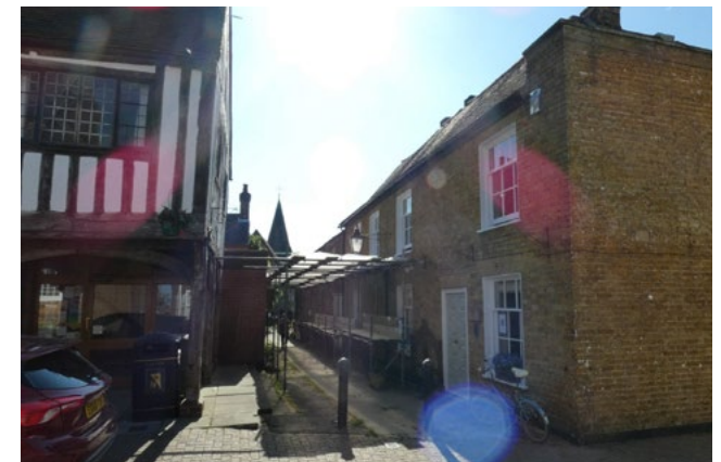
Fig 53. Old Market Hall adjacent to Mount House and its rear workshops with their potential for Local Listing and Grade I St Peter with St Paul Parish Church in the background.
