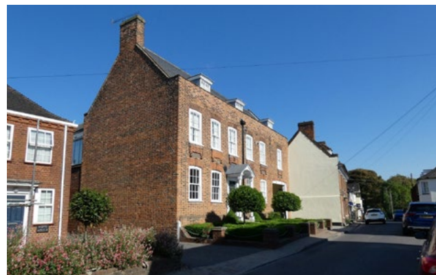
Fig 54. c18 Grade II* High House c14
