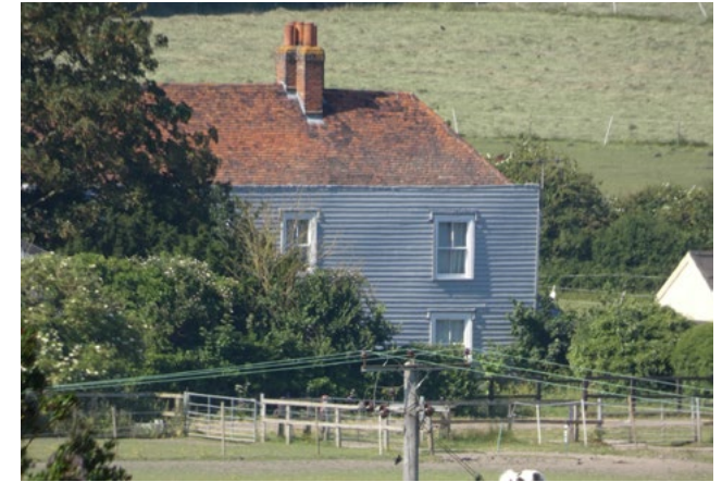
Fig 56. c18 brick-built Grade II listed Arden Hall
