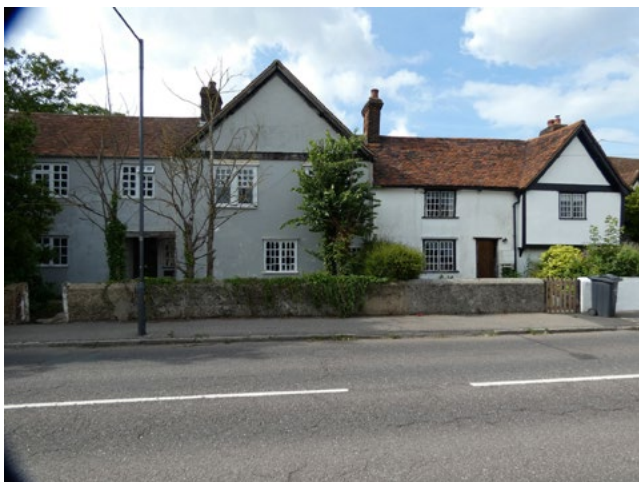
Fig 29. The property adjoining Laburnam Cottage does not appear to be listed and requires further investigation
