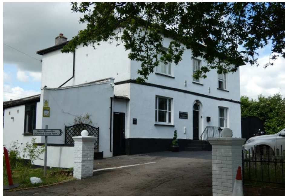
Fig 62. Grade II Listed Stifford Clays Farmhouse
