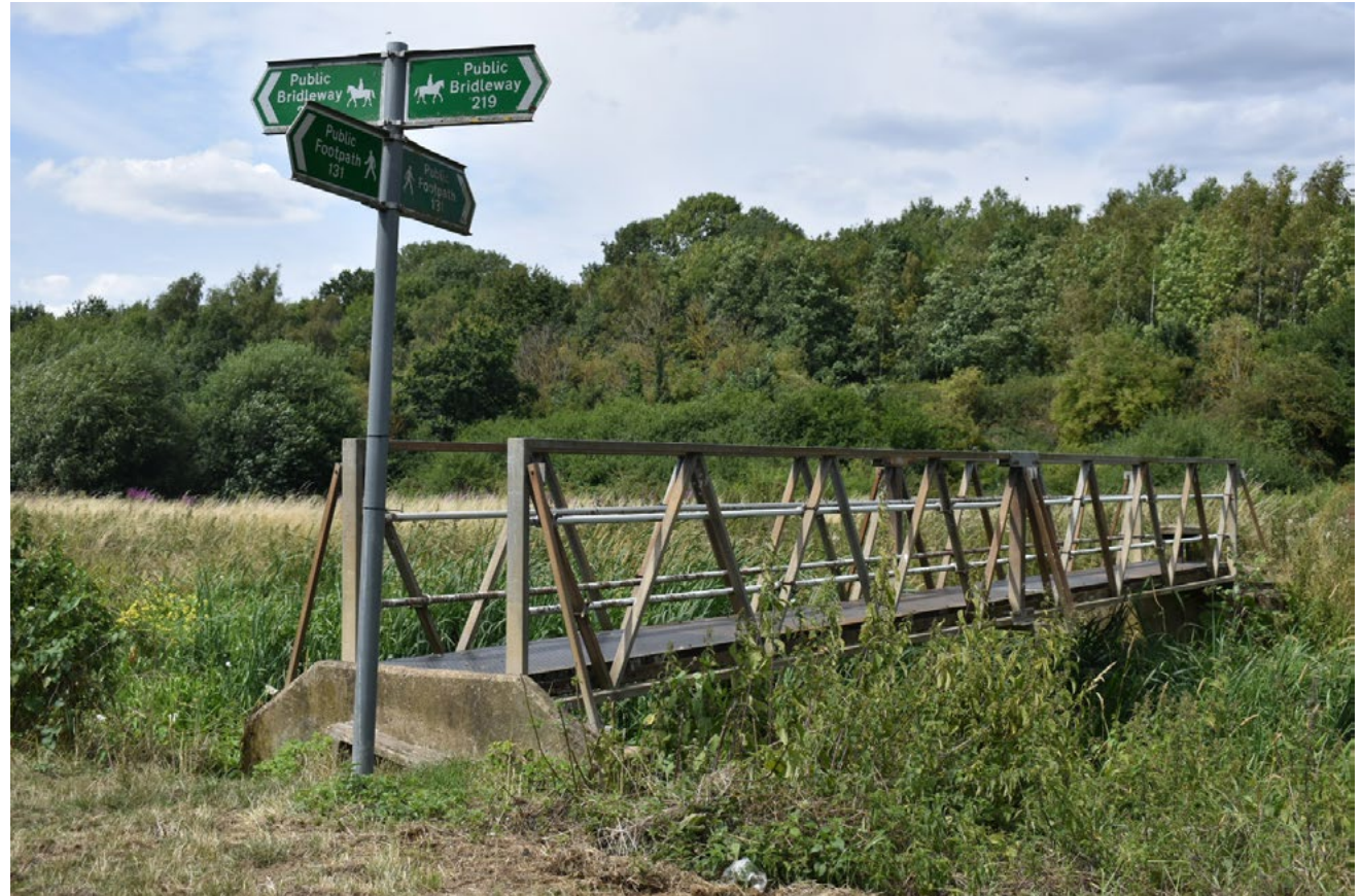
Fig 23. Footpath crossing the Mar Dyke
