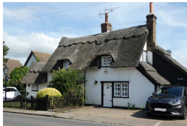
Fig 54. c17 thatched timber framed and brick cottages Caira and Fircot
