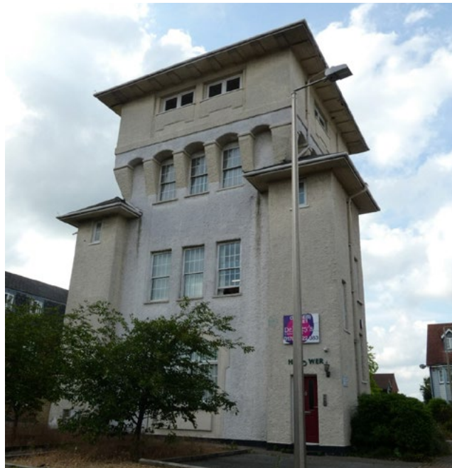
Fig 36. The original water tower from the former Stepney Children's' Home site
