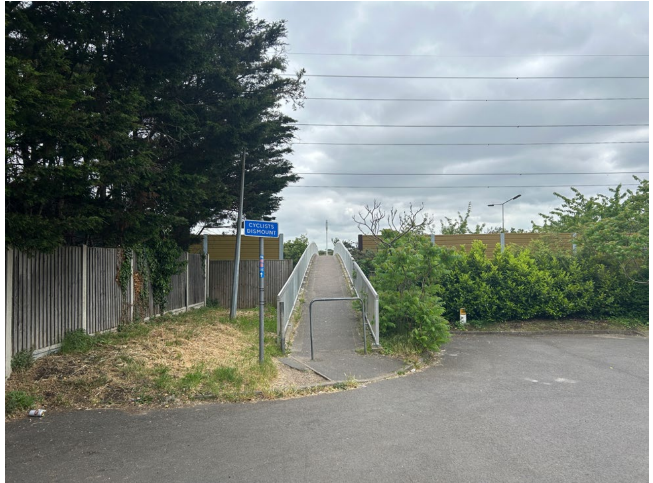
Fig 75. Pedestrian bridge to cross over the A13, south of the village
