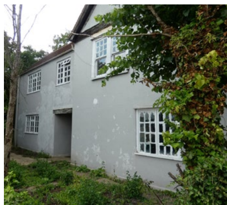
Fig 42. Western range of Laburnam, Middle Cottage & Old Post Cottage
