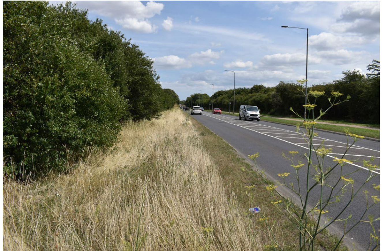
Fig 22. Enclosed views along A1306
