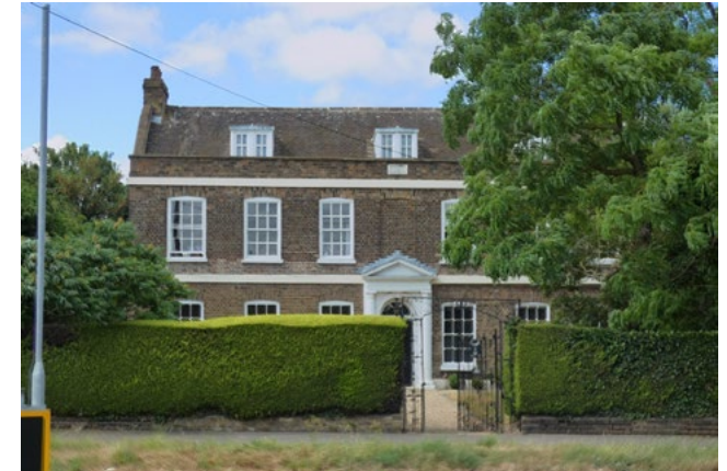
Fig 57. Grade II c18 brick-built Coppid Hall
