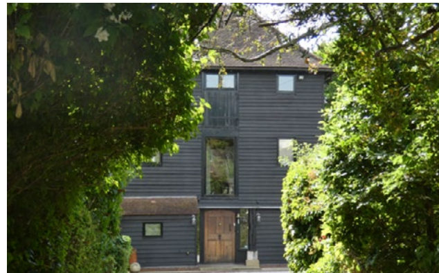
Fig 58. Unlisted timber barn behind Coppid Hall
