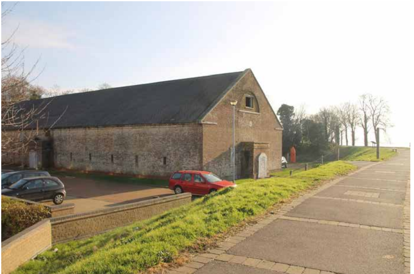
View 1: View looking southwards along the seawall to the Magazine building and beyond to the corner of the park and the Thames
