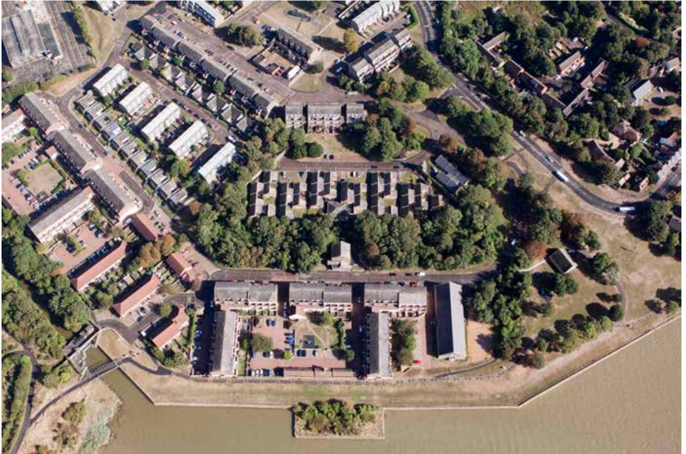
Figure 22: Aerial view of Purfleet Magazine looking north, showing its Thameside setting.
