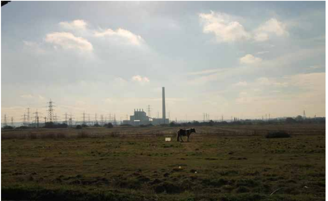
View 4: Looking south-west from the marsh edge towards Tilbury Power Station
