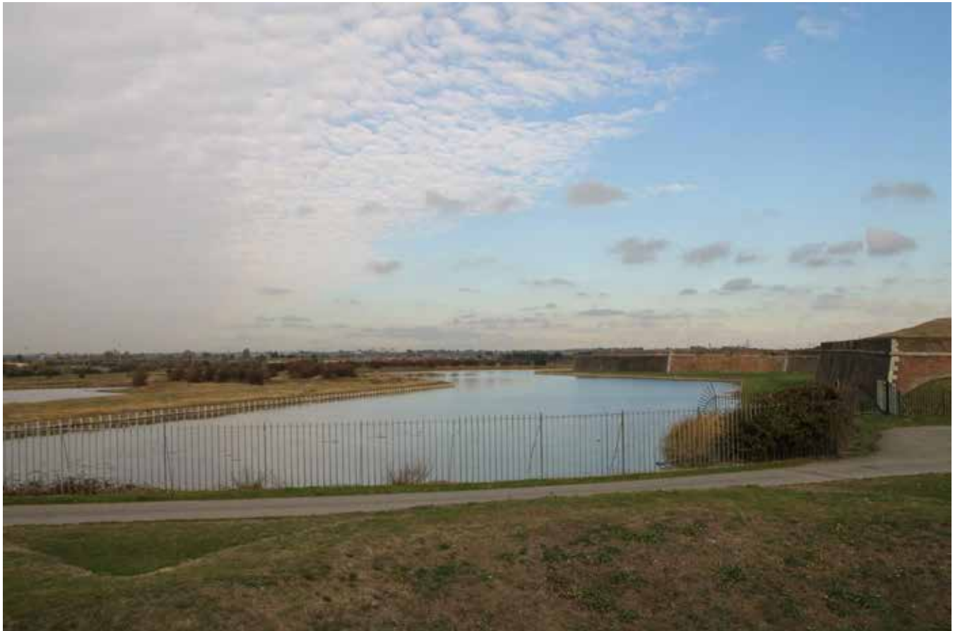
View 4: Looking north across the defensive moats to the wider marshland landscape to the rear of Tilbury Fort. The rooftops of modern Tilbury are just visible in the distance.
