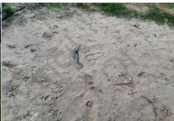
Finding: The sand safety surface is low and the membrane Action: Remove or resecure the exposed membrane and is exposed creating trip points
