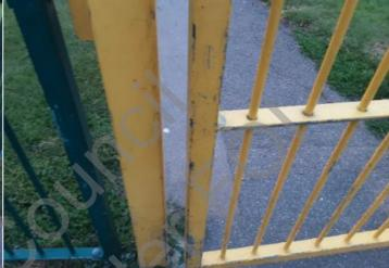
**Finding:** No slamming plate has been fitted to the gates and **Action:** Provide slamming plates the gate leaves pass the slamming posts
