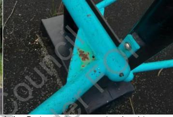
Finding: The paintwork on this item has been damaged or Action: Treat any rusting components and repaint worn exposing the metal underneath which is rusting
