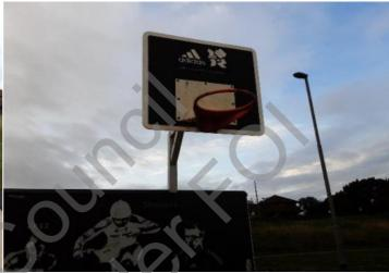
Finding: A clearly visible facility sign should be provided in a prominent position with the wording as detailed BS EN 15312- the equipment is not intended for children less than 3 years old- the warning - Do not climb on the framework or nets- the warning - Do not hang on the ring (if provided)- the warning - Do not wear rings or other jewellery- name and telephone number of the administrator- number to call in case of accident
