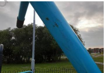
Finding: The paintwork on this item has been damaged or Action: Treat any rusting components and repaint
