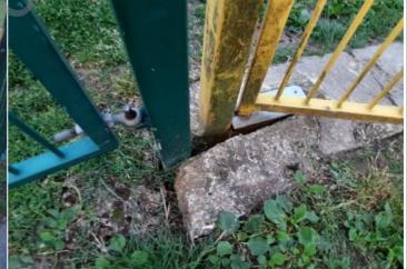
**Finding:** The concrete around the post has sheared and the **Action:** Reset the post post is loose in the foundations
