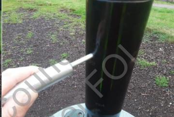
Finding: There is/are missing components creating finger Action: Replace the missing components entrapment/s in the redundant bolt holes and the item fails to meet the requirements of BS EN 1176 Part 1 4.2.7.6
