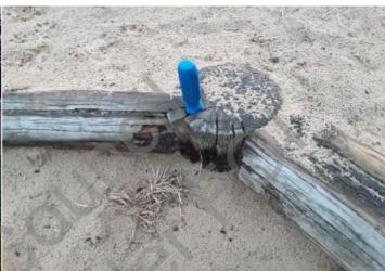
**Finding:** There are areas or parts of the timber edgings that **Action:** Replace all affected timbers have rotted or are missing
