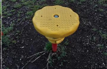
Finding: There is minor movement of the tops on the posts Action: Monitor
