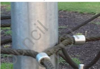
Action: Re-tension ropes to ensure the rope is spaced evenly around the post
