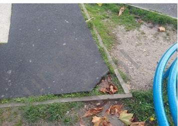
**Finding:** The surface is damaged and is lifting at the edges **Action:** Repair perimeter of surfacing to remove trip points and creating trip points
