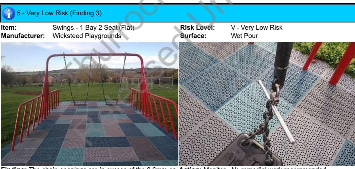
**Finding:** The chain openings are in excess of the 8.6mm as **Action:** Monitor - No remedial work recommended recommended by BS EN 1176
