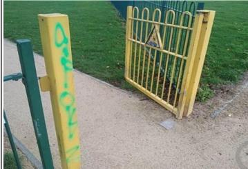
**Finding:** The gate is snagging on the surrounding surface preventing it from closing correctly
