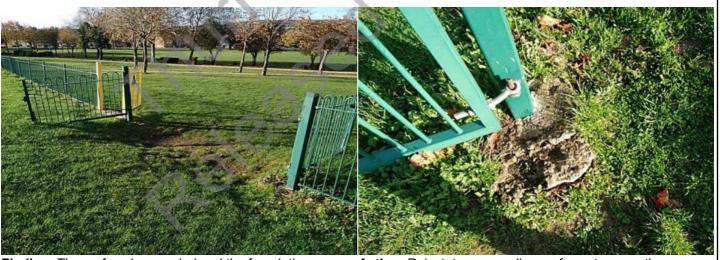
**Finding:** The surface has eroded and the foundations are exposed
