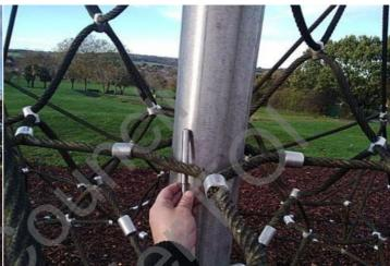
**Action:** Re-tension ropes to ensure the rope is spaced evenly around the post
