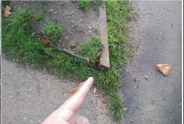
**Finding:** There are areas or parts of the timber edgings that **Action:** Replace all affected timbers have rotted or are missing
