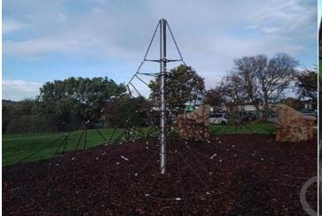
**Finding:** There is a potential crushing point between the rope and the central post in contravention of BS EN 1176 Part 1
