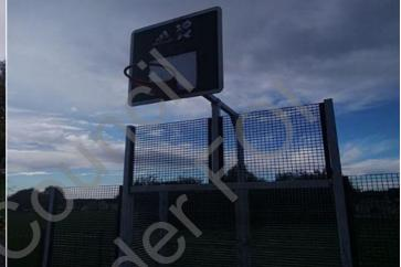
**Finding:** A clearly visible facility sign should be provided in a prominent position with the wording as detailed BS EN 15312- the equipment is not intended for children less than 3 years old- the warning - Do not climb on the framework or nets- the warning - Do not hang on the ring (if provided)- the warning - Do not wear rings or other jewellery- name and telephone number of the administrator- number to call in case of accident
