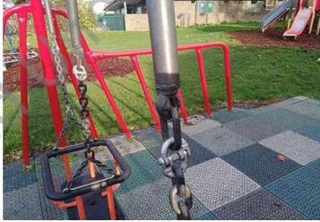
Finding: The connecting lugs are showing signs of wear
