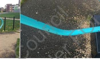
Finding: The paintwork on this item has been damaged or Action: Treat any rusting components and repaint worn exposing the metal underneath which is rusting
