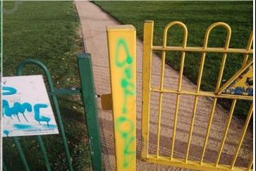
**Finding:** No slamming plate has been fitted to the gates and **Action:** Provide slamming plates the gate leaves pass the slamming posts
