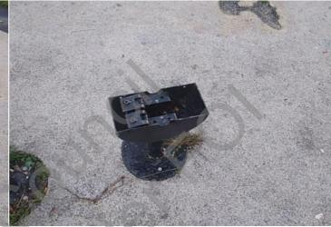
Finding: The mechanism has been removed from one item Action: Replace the missing components or remove the
