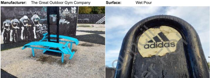
**Finding:** The signage is damaged and sharp edges are present
