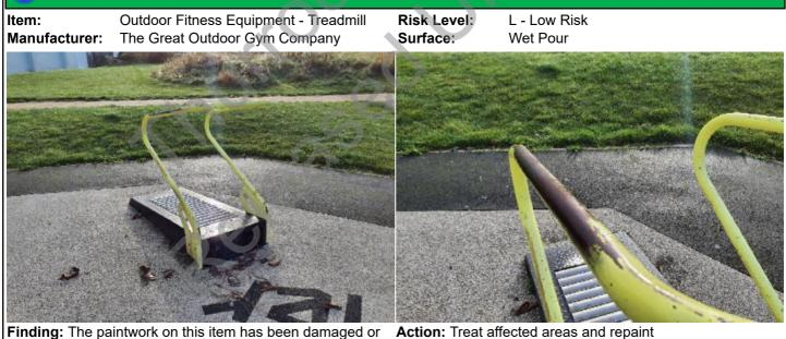
worn exposing the metal underneath which is rusting / corroding
