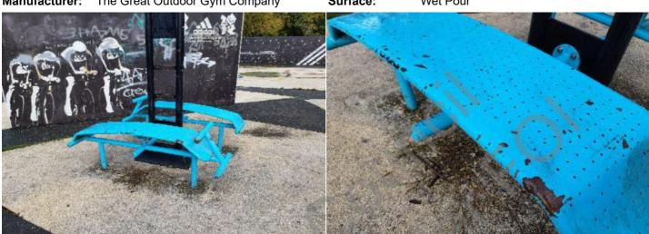
**Finding:** The paintwork on this item has been damaged or worn exposing the metal underneath which is rusting / corroding
