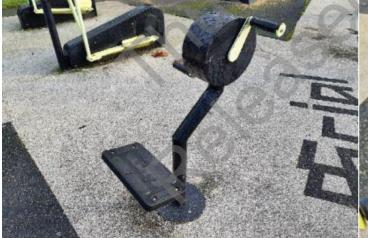
Finding: The paintwork on this item has been damaged or Action: Treat affected areas and repaint worn exposing the metal underneath which is rusting / corroding
