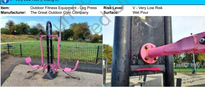
Finding: There is/are bolt cap covers missing or damaged on the item
