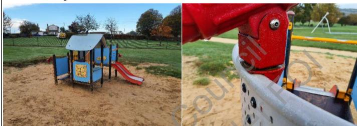
Finding: The paintwork on this item has been damaged or worn exposing the metal underneath which is rusting / corroding
