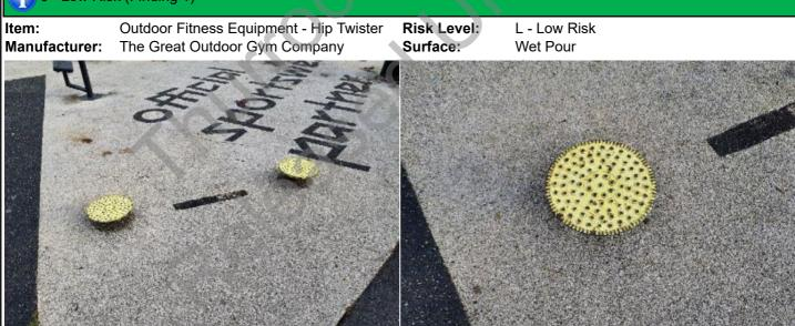
**Finding:** The rotating user station is not appropriately marked with a guideline of user direction and/or the original position as required by BS EN 16630
