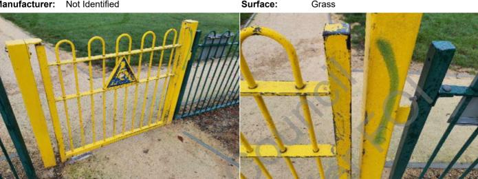
**Finding:** No slamming plate has been fitted to the gates and **Action:** Provide slamming plates the gate leaves pass the slamming posts
